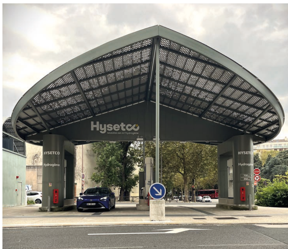
Refuelling station HySetCo - Porte de Saint Cloud - Paris
