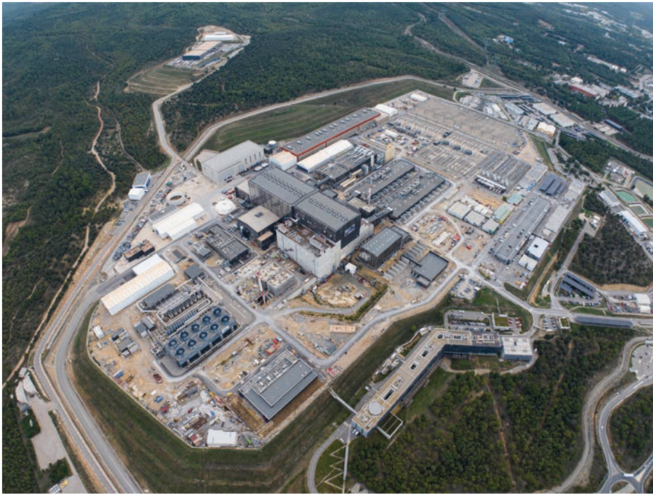
Aerial view of the ITER worksite in southern France
